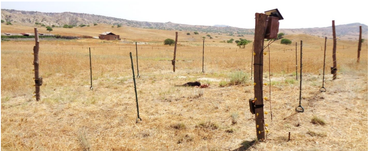
Figure37. Experimental electric fence installed in summer at Bugha-moedani
